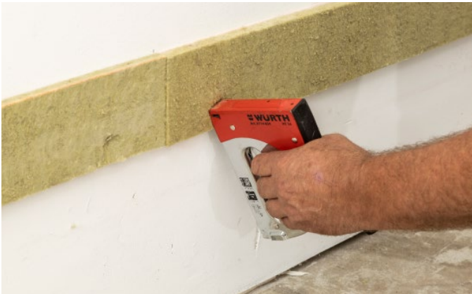
Bild 6: Wall fixing GIFAfloor edge insulation strips
