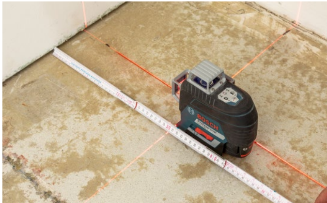
Bild 10: Measuring the wall connection element
