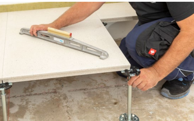
Bild 17: Levelling the raised floor elements
