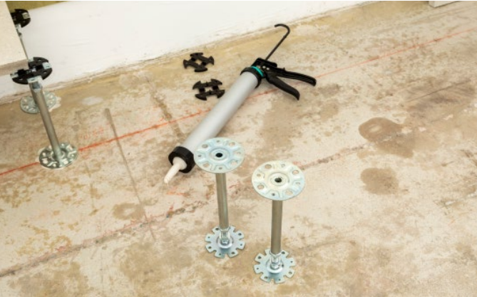
Bild 15: Positioning additional pedestals
