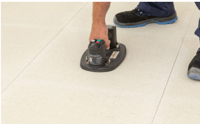
Bild 21: Re-seal raised floor with raised floor element
