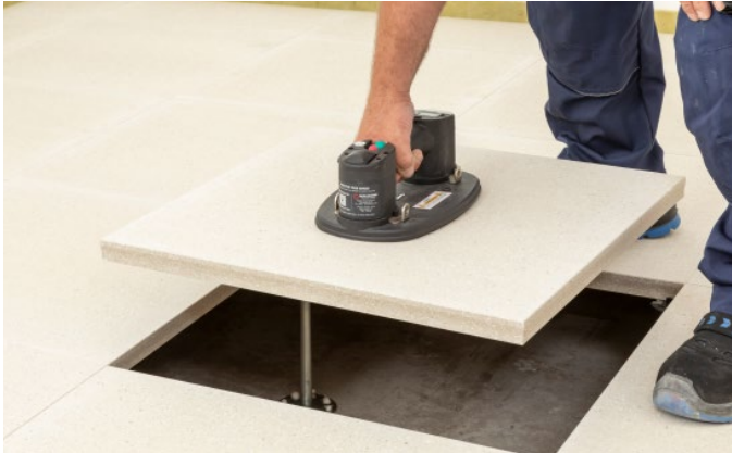
Bild 19: Lifting with vacuum lifting pad
