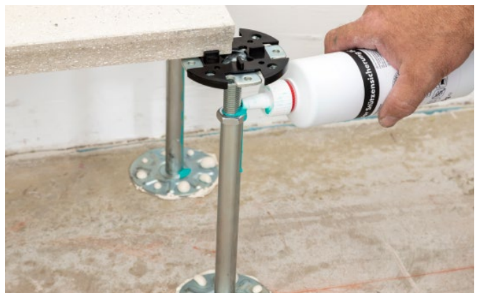
Bild 14: Installing the access floor element in the wall connection area
