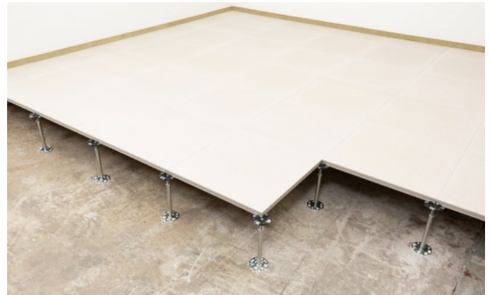
Bild 18: Installation of additional raised floor elements
